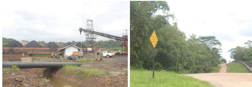
Figure 16. Mining and Excavation Activities at Teluk Dalam
