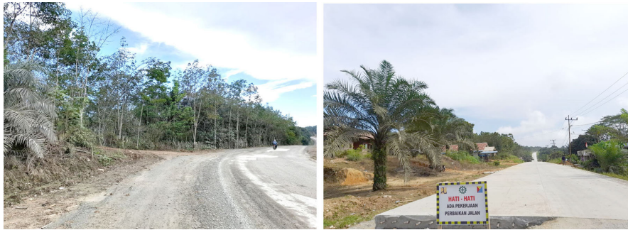
Figure 14. Road Construction at the Location of IKN (Photo credit: Hilary Reinhart)
