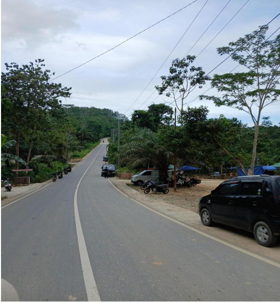
Figure 1 The connecting road between Maridan and Riko sub-districts, which has been repaired and widened (Photo by Muhammad Yuda Aditya, 2025).
