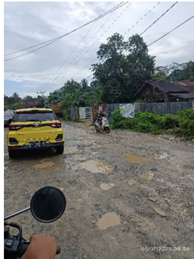
Figure 14 Potholed road on the border of Sepaku Village and Bukit Raya Village (Photo by Maulidia Savira Chairani, 2025)
