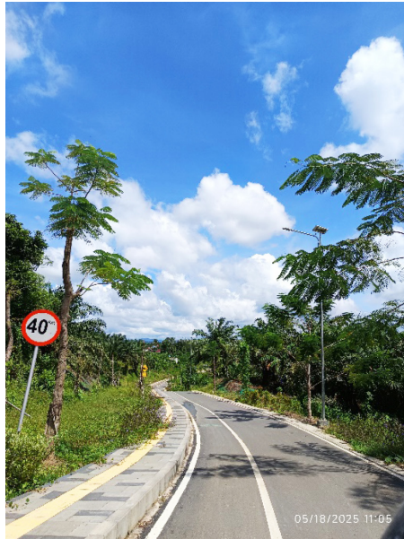
Figure 23 Inspection Road of SPAM (Source: Authors, 2025)
