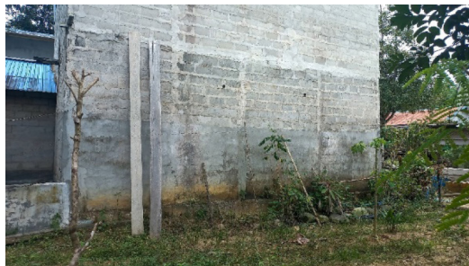
Figure 17 Flood marks on one of the walls of a community house (Photo by: Moh Syahrul Irfan Fahmi, 2025)
