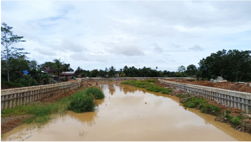
Figure 14 Construction of Tiles for Sepaku River Normalisation (Source: Authors, 2025)
