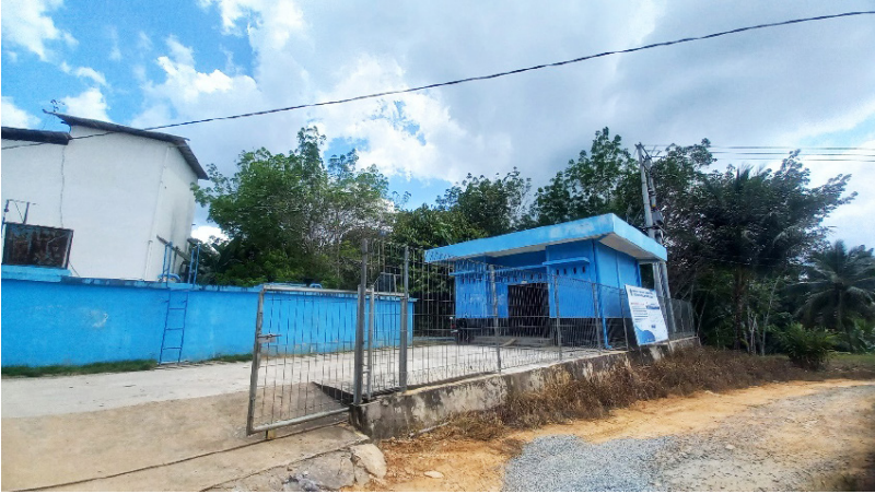
Figure 27 Maridan Village Water Supply Company (Photo by: Moh. Syahrul Irfan Fahmi, 2023)
