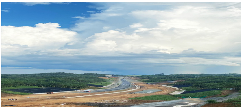
Figure 19 The development of highways to support IKN (Photo by: Adji Saiddinullah, 2025)
